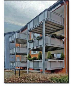
In thicknesses of 20, 25 and 35 mm, the balcony slabs are available with a general building approval (Z-10.9-47 | until 2023).
